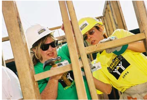
A Crew Leader teaches a homeowner how to install blocking
